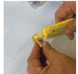
Apply gas pipe sealant all the way around the Flair Adapter's thread that will connect to the Natural **Gas Valve**
