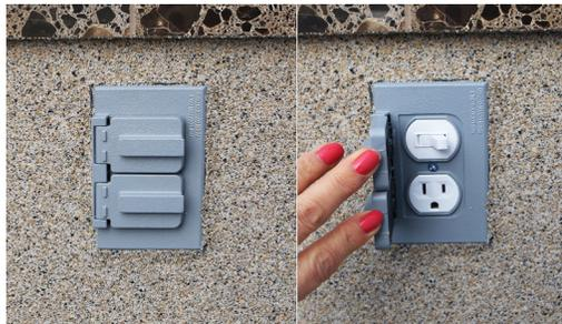
This switch/outlet combination is shown closed (left) and open (right).
