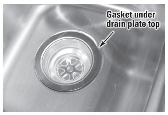
b. Hold the drain plate bottom in place and insert the drain pin connector. Tighten in place using a coin or a washer. Center and adjust as needed.
