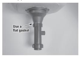
Attach trap (6) to drain. 7.
