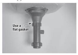
Attach trap (6) to drain. 7.
