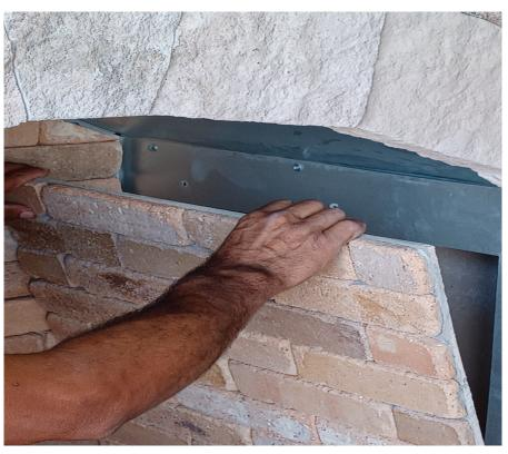
Once you successfully remove the screws, you will be able to carefully tilt the side panel forward.
