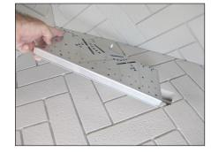
2. Remove the right side refractory wall from the fireplace by removing the 4 screws.
