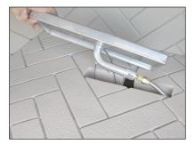
5. Reach through the gap in the open right side and pull the flex line and black sparker wires.
