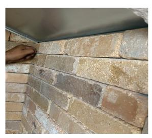
The picture to the left shows one of the screws without the plastic bushing.
